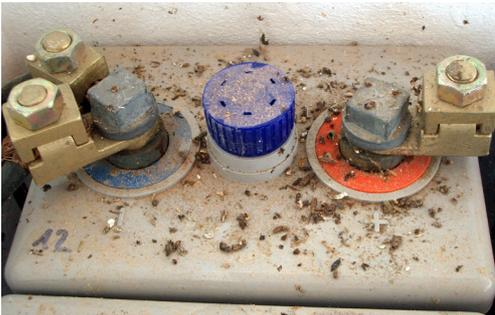
**Figure 5:** New battery after a couple weeks: rats liked the place, leaving excrements.
